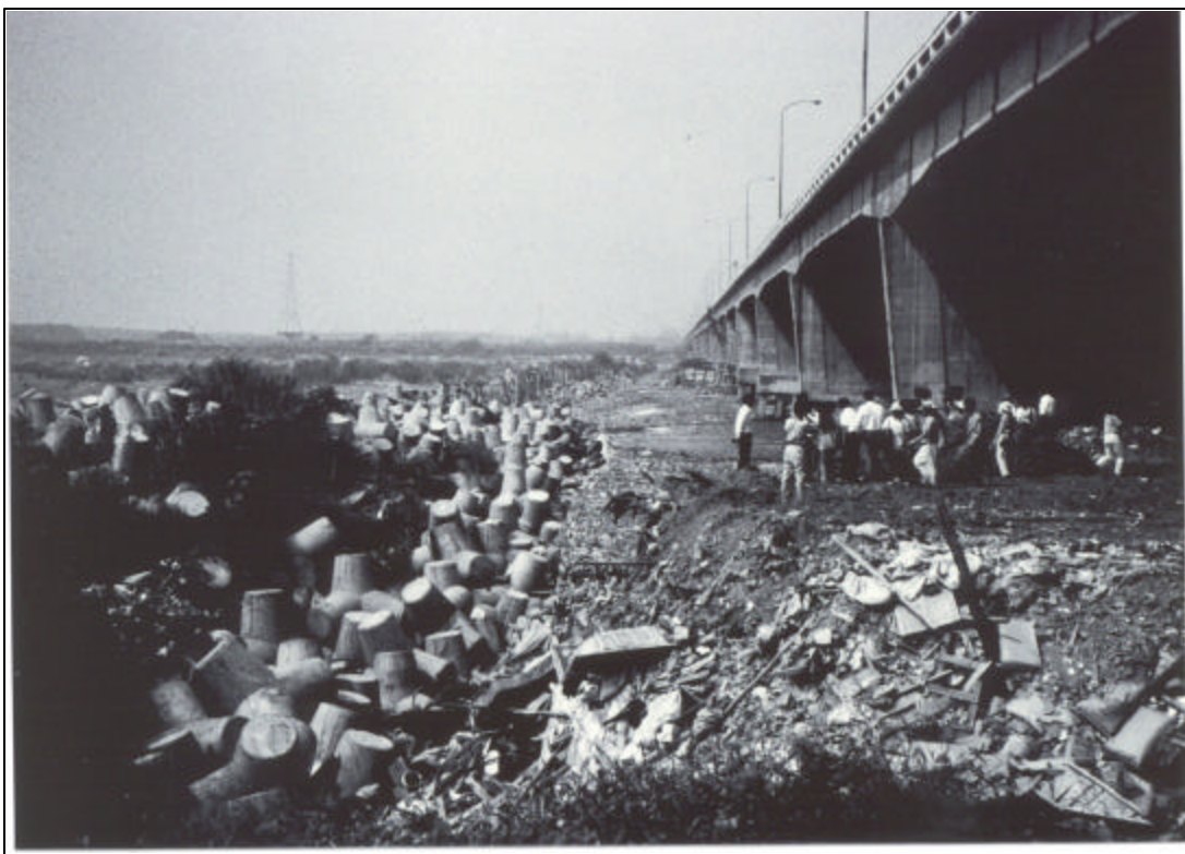
Figure 29. Undercutting and grade control efforts along the downstream side of the Kaoping Bridge over the Kaoping River, Taiwan, to control incision caused by massive gravel mining downstream (Photograph by Kondolf, October 1995).
