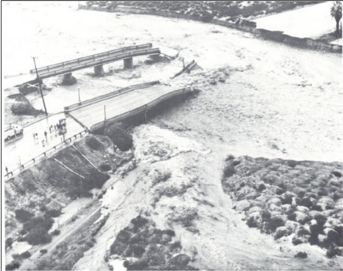
Figure 42. Collapse of Foothill Ave Blvd during the flood of 1969 in Tujunga Wash, Los Angeles (Source: Scott 1973).
