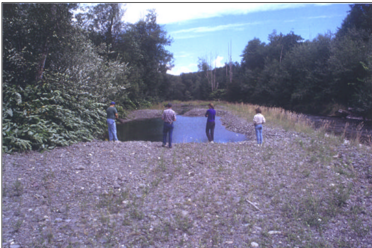
Figure 46. View downstream to gravel trap in a left bank gravel bar on the Big Quilcene River (Photograph by Kondolf 2001).
